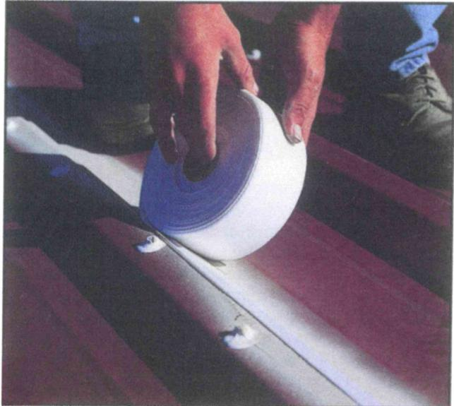
Reinforce existing seams with Spunflex<sup>®</sup> or Butyl Tape and base coat
