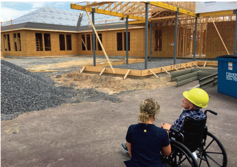
Construction on the addition at Heritage Springs Memory Care, Lewisburg, is well underway! Pictured is the 'Resident Construction Manager' checking in on the progress. The new 28-bed neighborhood is expected to open this winter.
